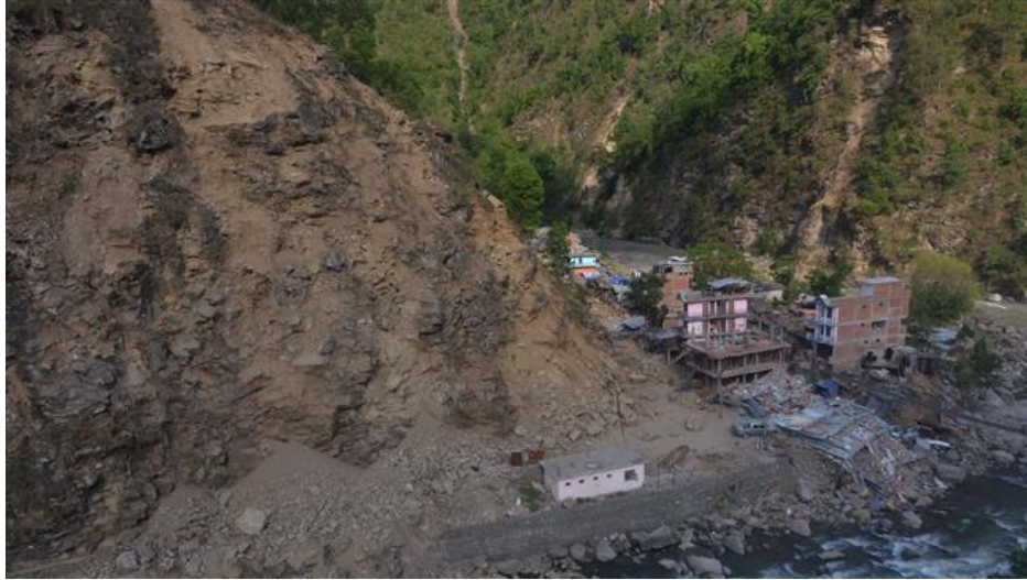
Image 2 – Resultant Landslide from the Earthquake 9
